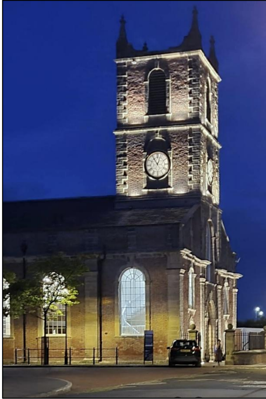
Tower from the North.
